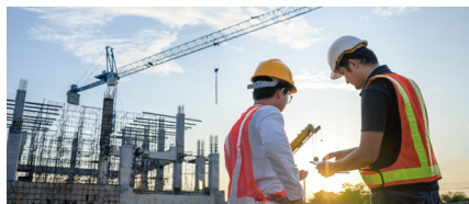
Mines and construction sites
